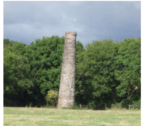
Old chimney near Minehouse Farm
